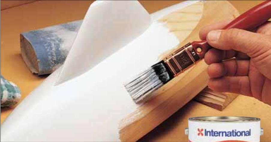
Quick-drying, alkyd, resin-based undercoat.
